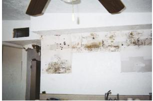
Just because you don't see it doesn't mean it isn't there. While no mold is visible on the wall, removing the cabinets tells a different story.
